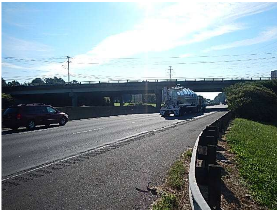
LOOKING NORTH AT APPROACH ROADWAY
