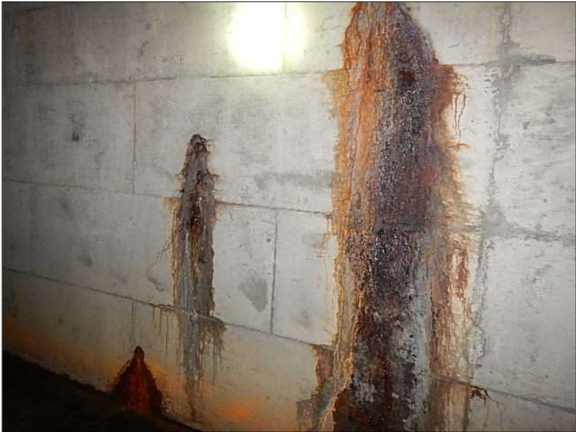
RANDOM CRACK WITH EFFLORESCENCE AND RUST
