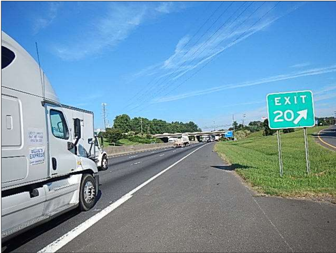
LOOKING SOUTH AT APPROACH ROADWAY
