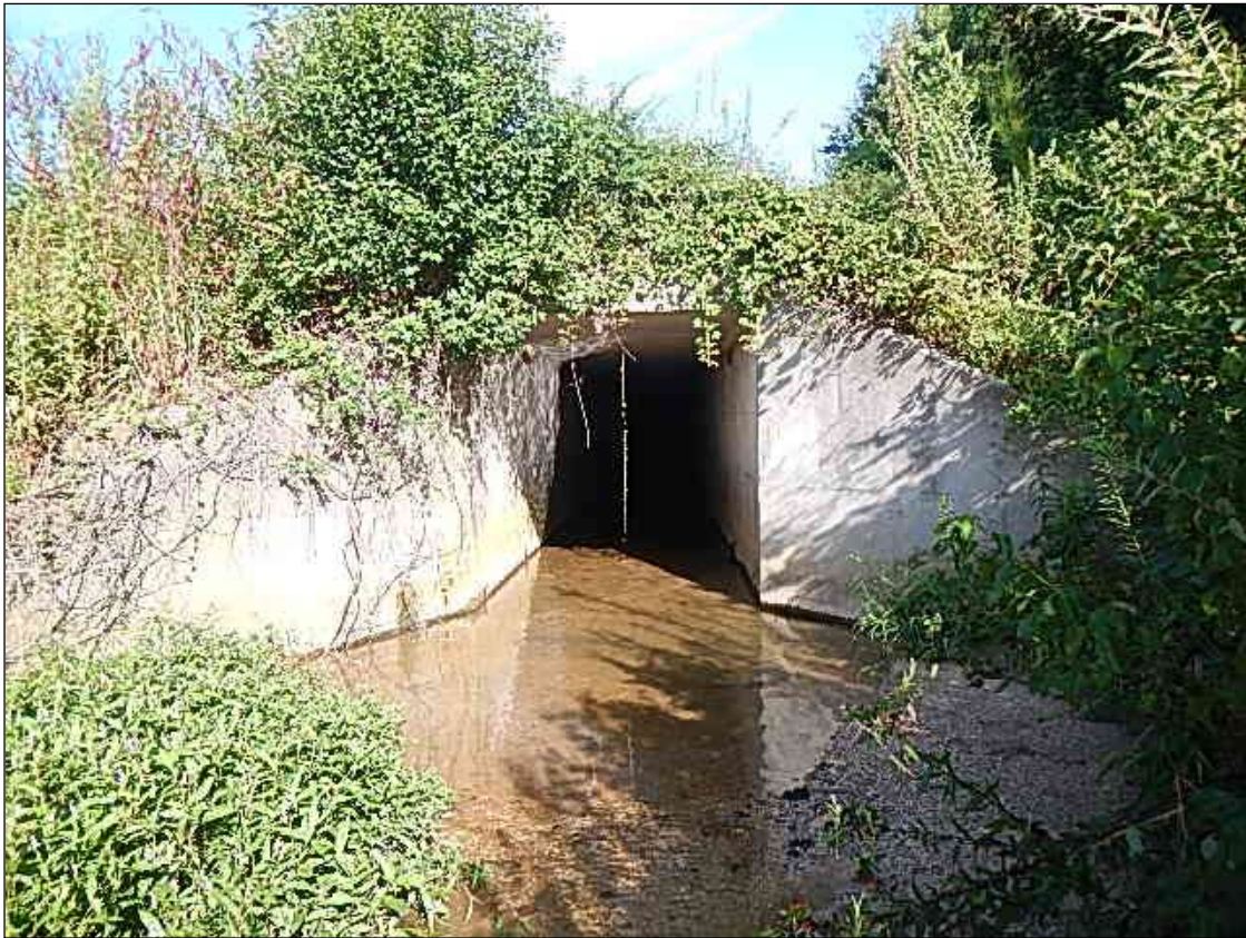
LOOKING EAST AT OPENING
