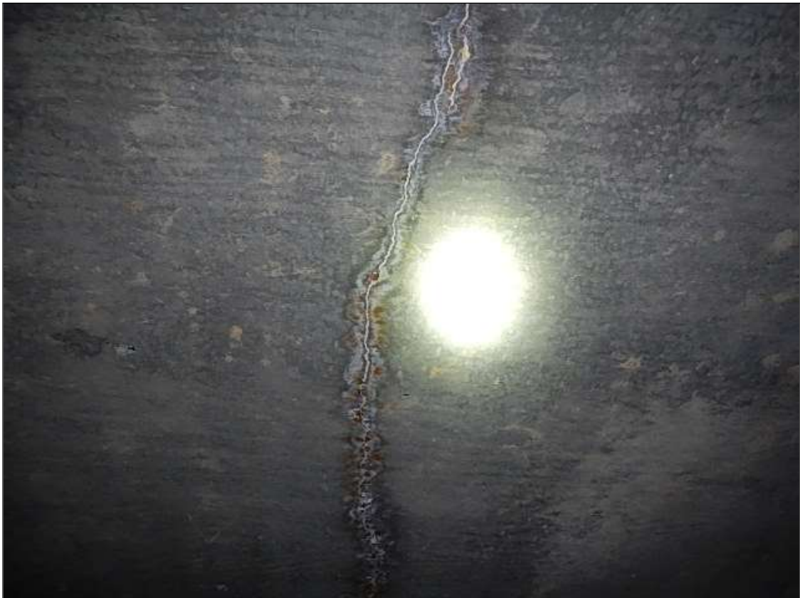
RANDOM CRACK WITH EFFLORESCENCE
