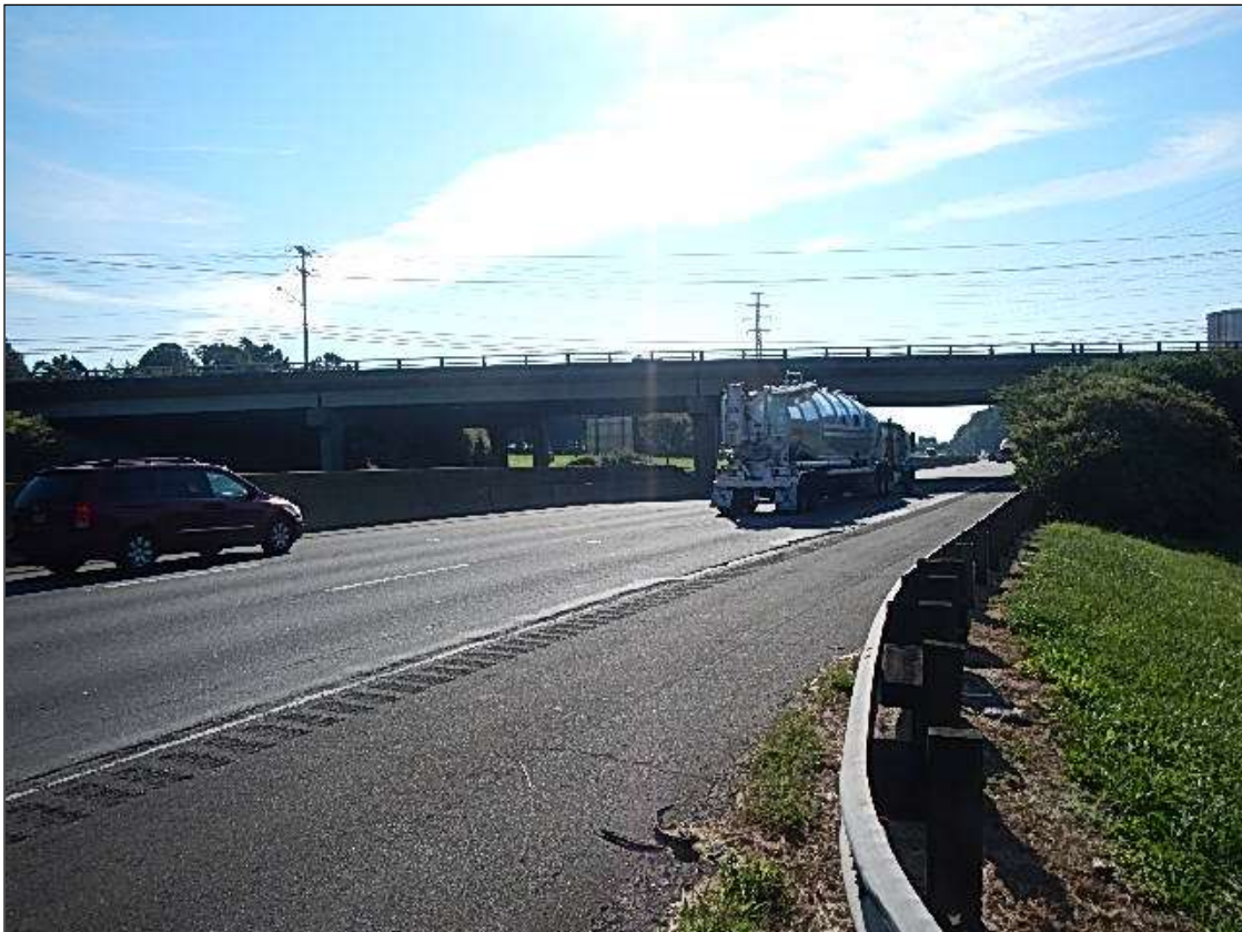
LOOKING NORTH AT APPROACH ROADWAY
