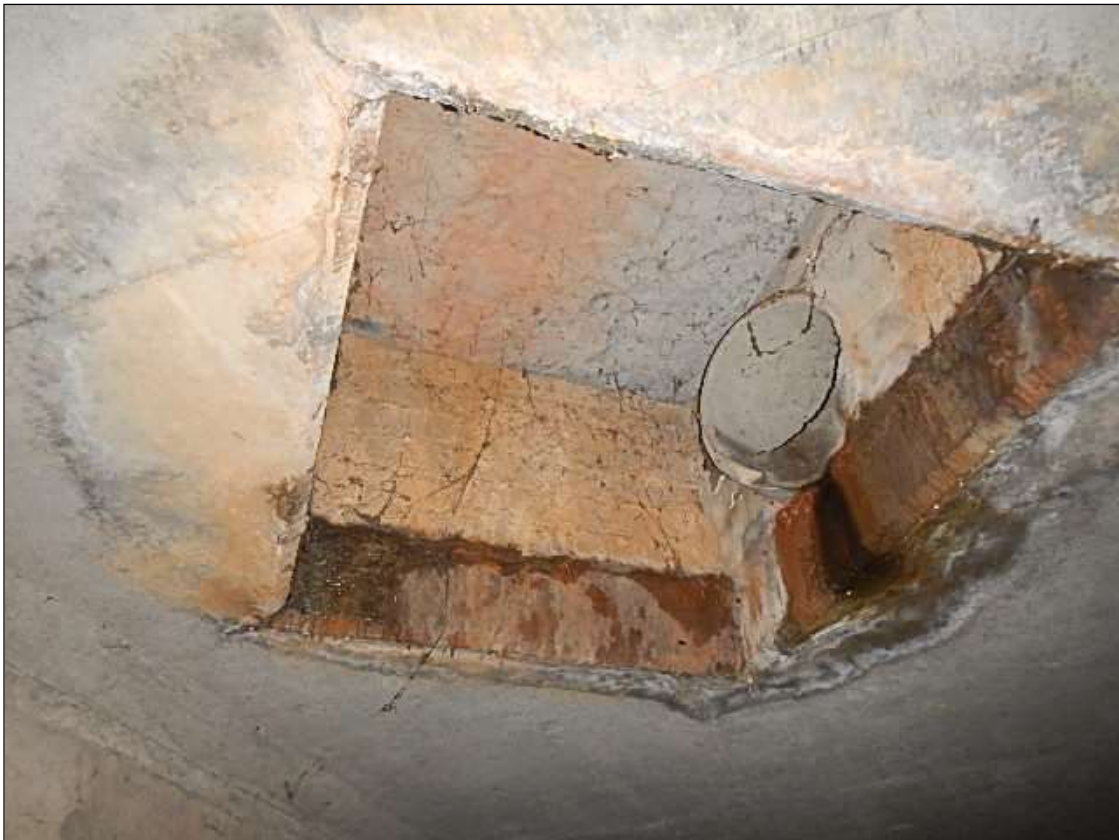
TOP SLAB NEAR EAST OPENING
