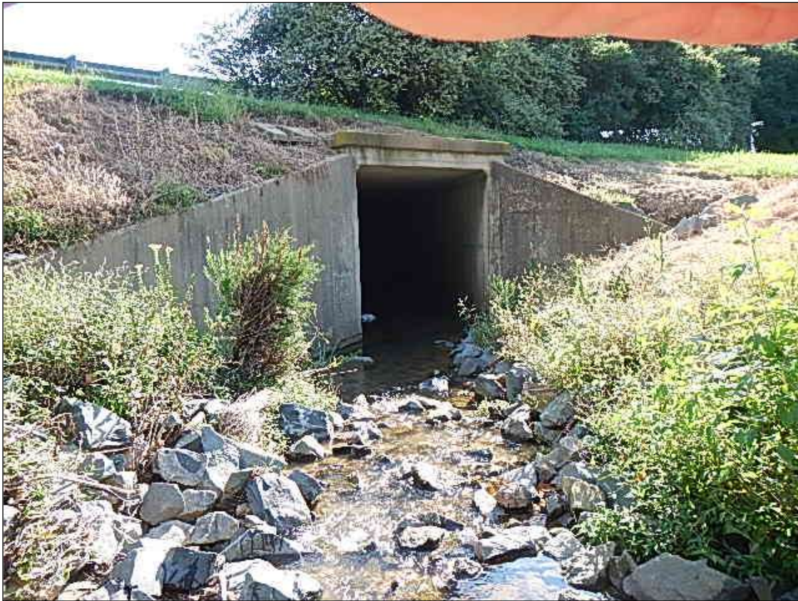
LOOKING WEST AT OPENING
